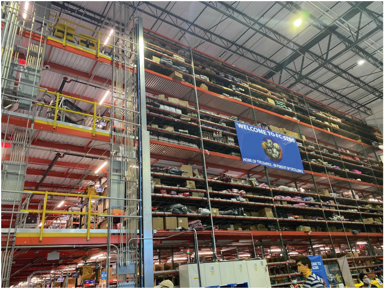
Figure 5: The Pick Module included 1.1 million square feet of floor area on 4 levels.
